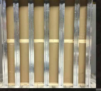
Another advantage is that StoneAdvise America offers benefits in terms of logistics, as the mounting of the underlying structure can be 'separated' from the subsequent attachment of the cladding panels.
